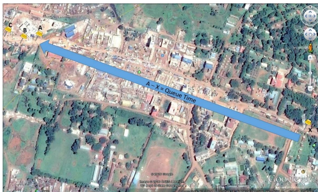
Figure 7.2: Aerial View of OSBP and the Positioning of the Enumerators
