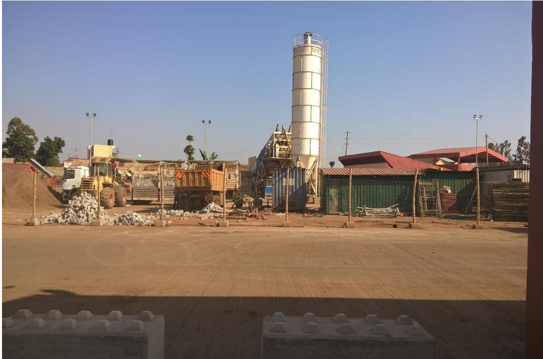
Figure 2.6: Busia - Uganda: Truck Parking Area occupied by Construction Works
